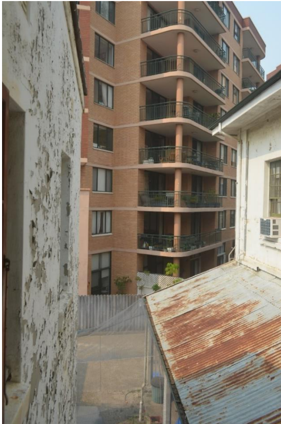
Figure 5: Neighbouring residential flat building, viewed from the subject site looking south
