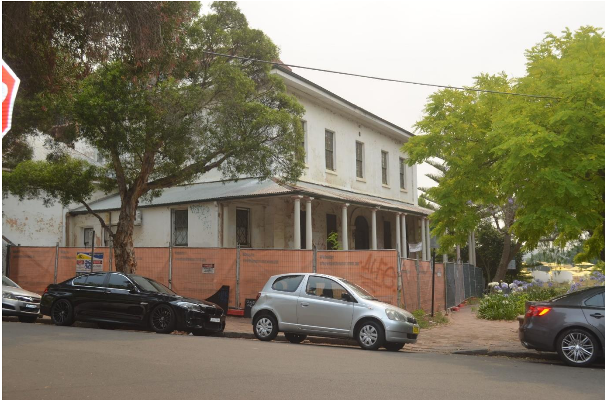
Figure 3: Site viewed from Buckingham Street, looking west towards Bedford Street
